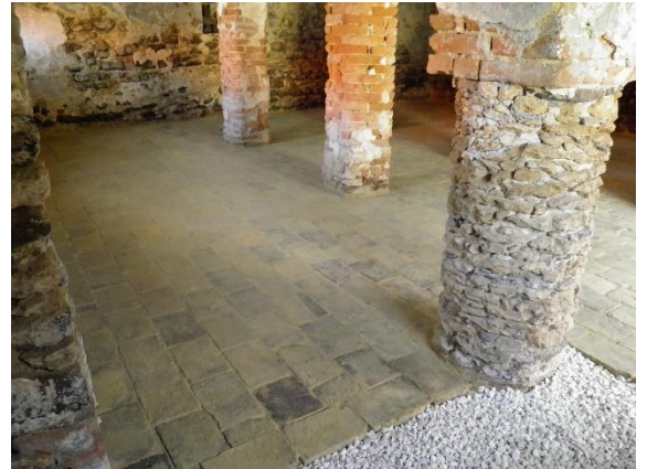
Figure 10 The pavement and columns
