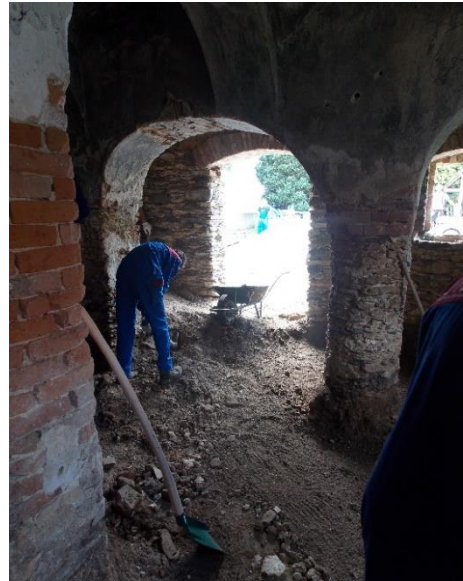
Figure 7 Carrying out the enclosure substrate
