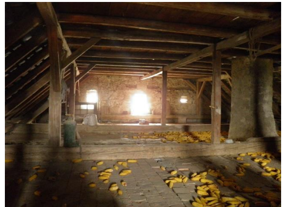
Figure 11 The attic of the house
